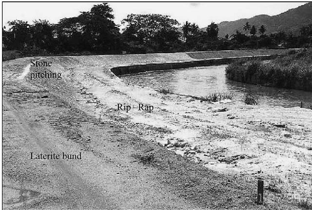
Fig. 7. Stabilization of Pari River after 1997 flood.
