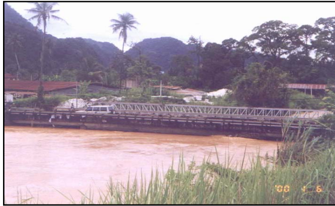
Figure 3: Water Level (45.950 m) at Kampong Tanjung Bridge During 1999 Flood Event (DID Kinta/Batang Padang, 2002).
