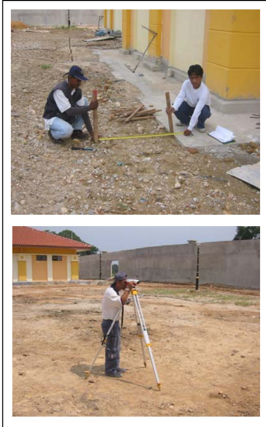
Figure 7 Setting out works.
