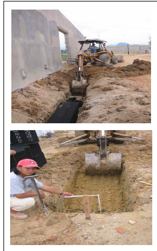
Figure 8 Excavation works and invert level checking.
