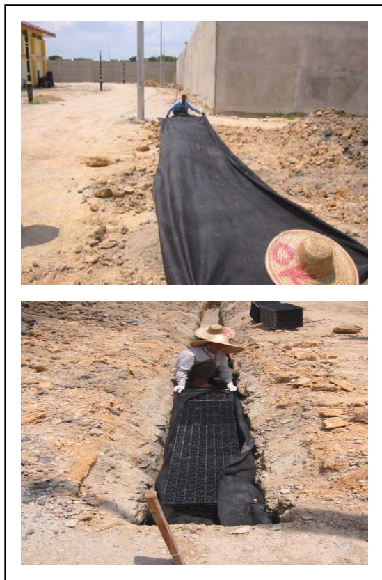
Figure 10 Installation works of subsurface module.
