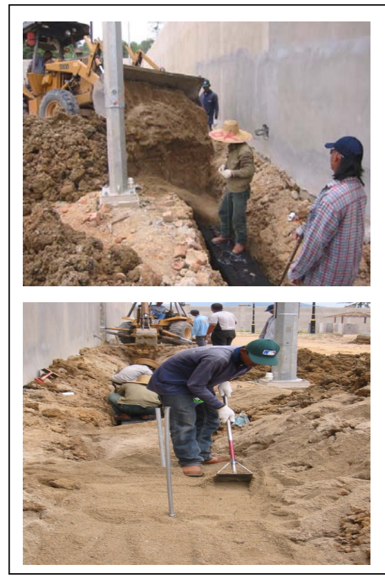
Figure 11 Sand Backfilling works.
