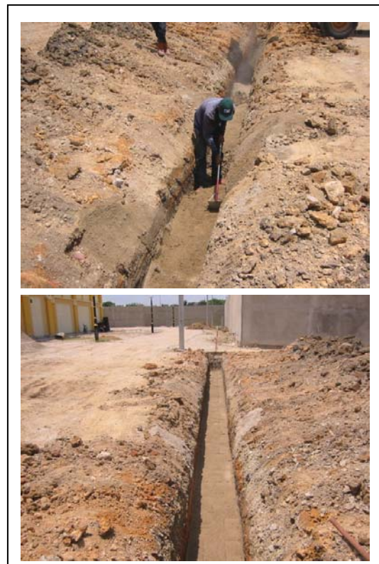
Figure 9 Sand bedding laying.
