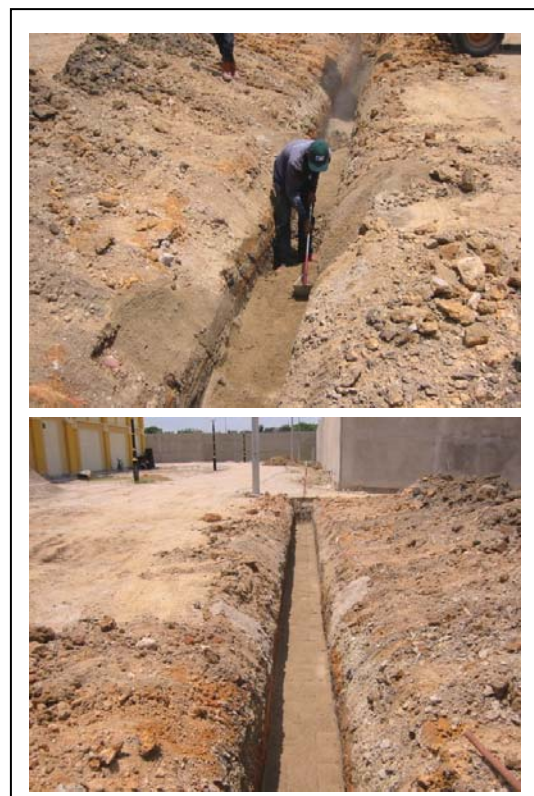
Figure 9 Sand bedding laying.
