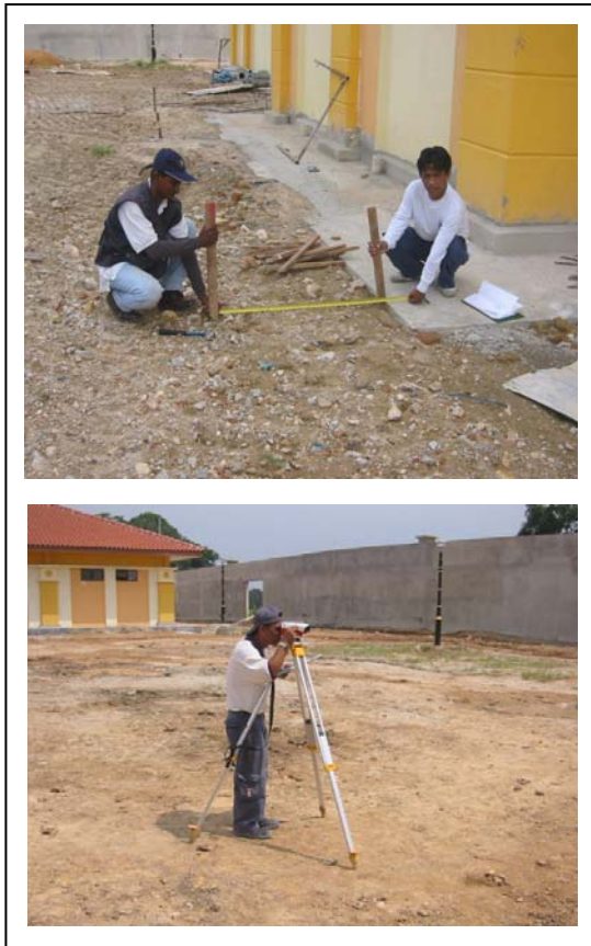
Figure 7 Setting out works.
