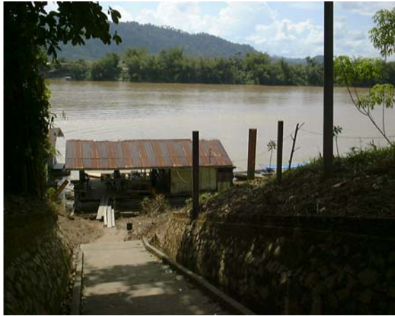
Figure 5 The “Tangga Krai” a flood warning structure.
