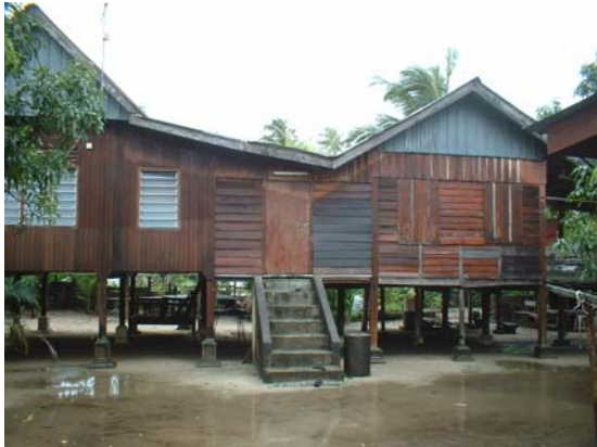
Figure 3 The traditional Malay house is a good example of a flood-proof structure.
