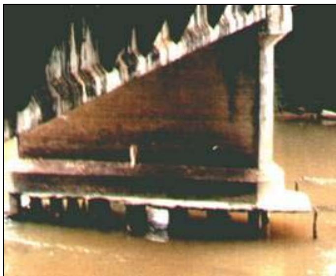
Figure 2 Bridge Crossing Ketil River (1km Upstream of Muda River)
