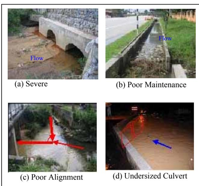
Figure 4 Current Conditions of Existing Berop River and Contributing Drainage System
