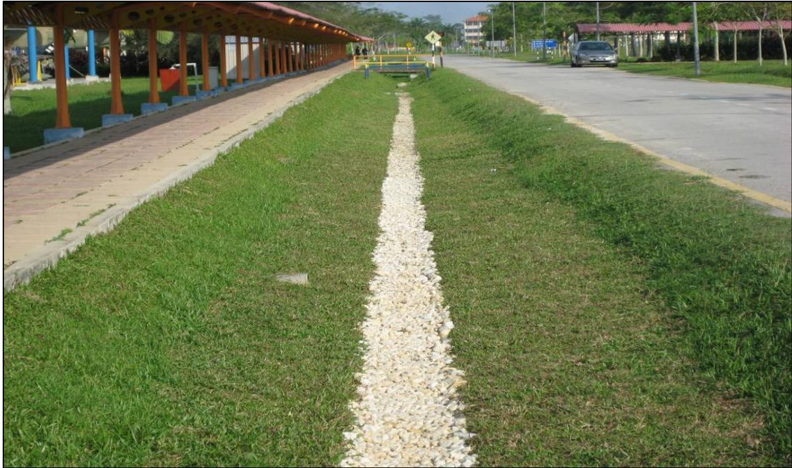
**Figure 2.** An ecological swale with river gravels making up the low flow channel.
