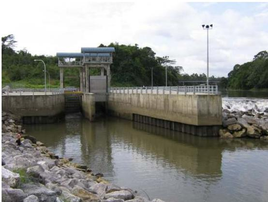
(a) Lock and Sediment Sluice
