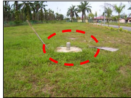
Figure 4 : Well 1 in RECESS area
