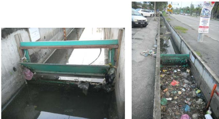
**Figure 7** Litter caught at the gate preventing the gate to close properly (left); accumulation of debris behind the gate during in between period of gate operation (right).
