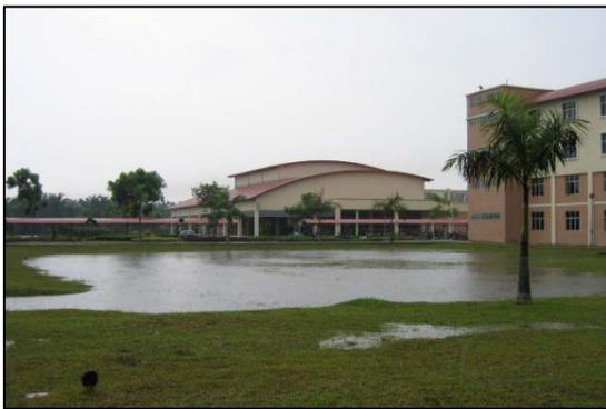
Figure 3: Constructed Dry Pond (after Storm Event)
