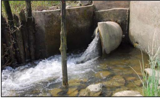
Figure 9: Check valve used to provide flow in one direction only through a culvert
