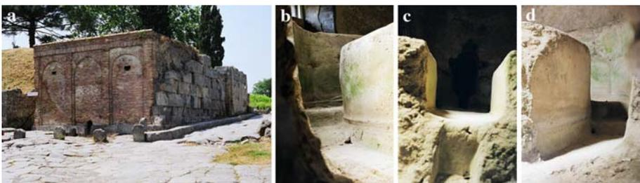
**Fig. 9** *Castellum divisorium* in Pompeii. (a) Building housing the *castellum*. (b–d) Three gated channels of the *castellum* used to control flow to geographical areas of Pompeii (photos copyright by L.W. Mays)
