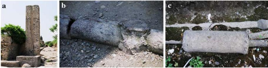
**Fig. 10** Components of water distribution system in Pompeii. (a) Water tower (secondary *castella*) with a storage tank was mounted on top of the tower. Lead pipes were used for the flow of water to and from the tank and were placed in the vertical recessed portion on the tower. The exiting pipes (*calices*) branched off to supply various customers and public fountains. (b) Lead pipe and joint found along the street. (c) Junction box. (photos copyright by L.W. Mays)
