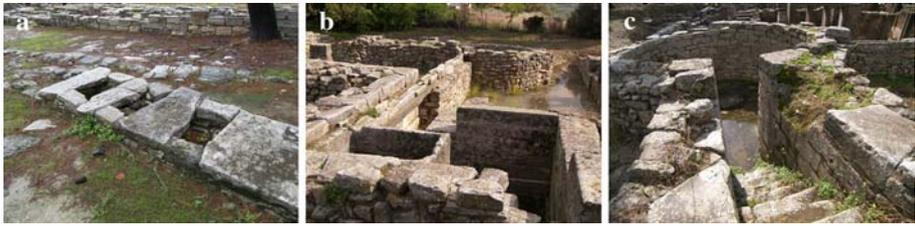
**Fig. 3** Water system in Tyliisos, Crete. (a) Aqueduct bringing water from springs. (b) Sedimentation tank in foreground with stone channel connecting to cistern. (c) Steps leading down to cistern (photos copyright by L.W. Mays)
