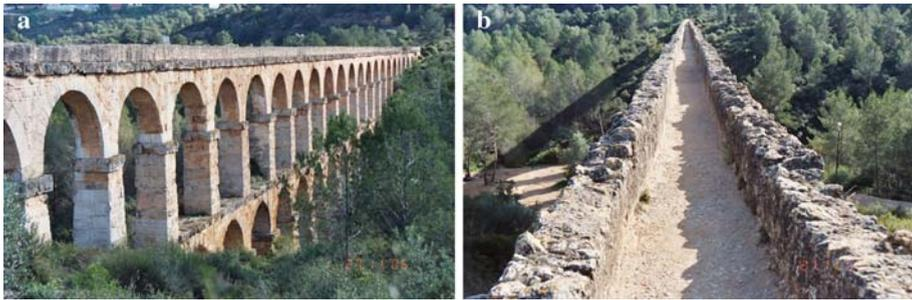
**Fig. 7** Aqueduct bridge of Ferreras (known as Puento del Diablo (devil's bridge) near Tarragona, Spain built during the first Century BC. Aqueduct bridge is 217 m long and 27 m high. (a) Bridge consists of two tiers of arches with diameters of 5.9 m (20 Roman feet) with a 15 cm variation and a distance between centers of piers of 7.95 feet (26 Roman feet). (b) The *specus* has a modern day width of 2.5 Roman feet (photos copyright by L.W. Mays)
