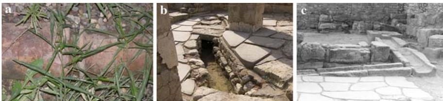
**Fig. 2** Water components in Knossos. (a) Pipes made of terracotta. (b) Drainage channel. (c) Carved stone elements of rainfall harvesting system collecting water falling from roof (photos copyright by L.W. Mays)
