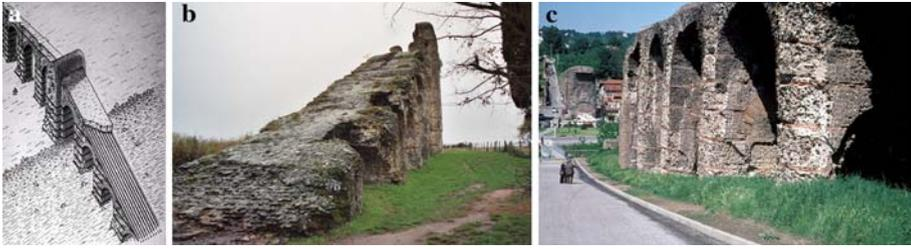
**Fig. 8** Siphon of aqueduct of Gier, Beaunant, France near Lyon (Ancient Lugdunum). (a) This reconstruction shows ramp with header tank on the top and the nine lead pipes of the siphon [23]. (b) Ramp of the siphon near Chaponost (photo copyright L. W. Mays). (c) The *venter* bridge of the siphon near Beaumont (Courtesy Henning Falhbusch)
