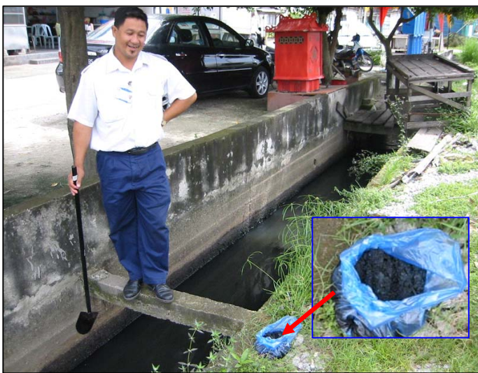
Figure 9 Sedimentation in Trunk Drain. (MPSP, 2004)
