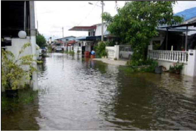
Figure 4. Main access road in the Study area was flooded. (MPSP, 2004)
