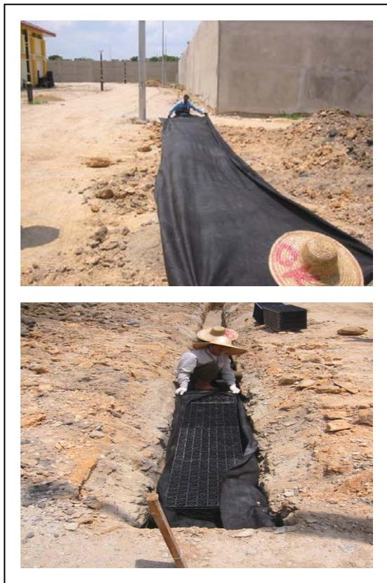
Figure 10 Installation works of subsurface module.
