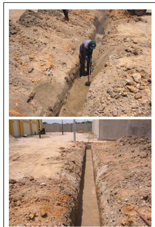
Figure 9 Sand bedding laying.
