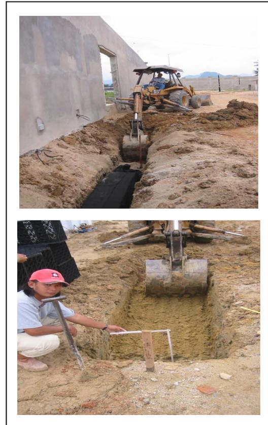
Figure 8 Excavation works and invert level checking.
