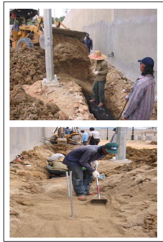
Figure 11 Sand Backfilling works.
