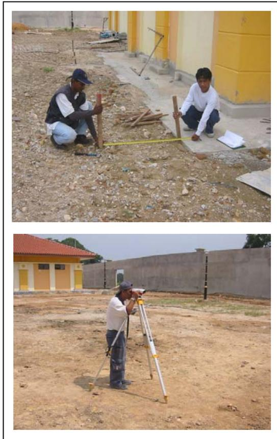
Figure 7 Setting out works.
