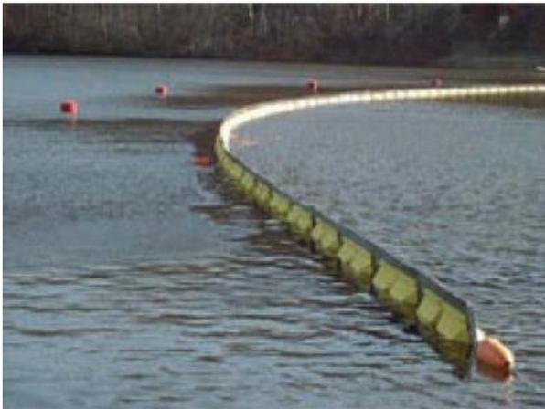
Figure 11 Flexible boom intake
