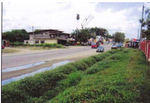
(a) No maintenance on main drains
