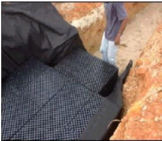
c) Online subsurface detention
