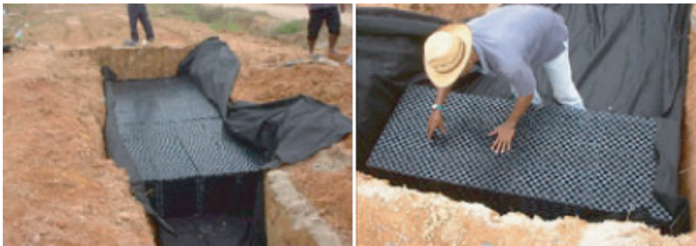
Figure 21 Modular subsurface detention.
