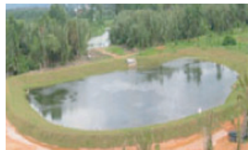
Figure 25 View of detention pond.
