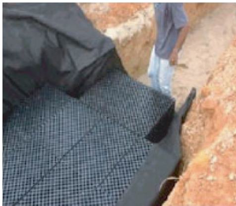
(c) Online subsurface detention
