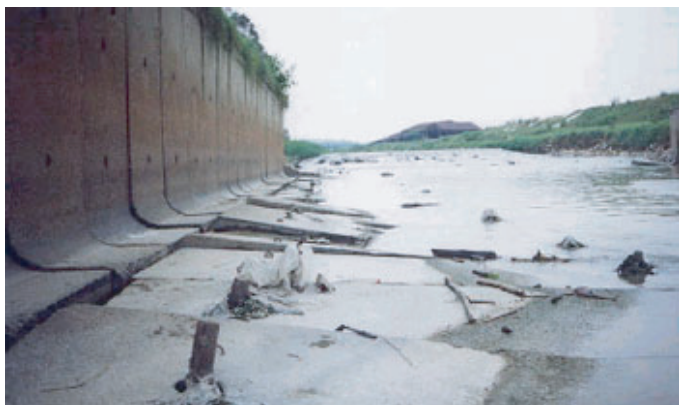
Figure 3 Typical channel erosion due to increase of discharges in the river channel (Pari river, Ipoh).
