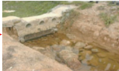
Figure 20 Ecological swale Type C (outlet).
