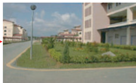
Figure 14 Typical view of perimeter swale.
