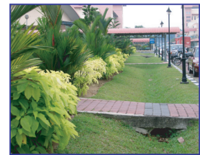
GS4 (Perimeter swale)
