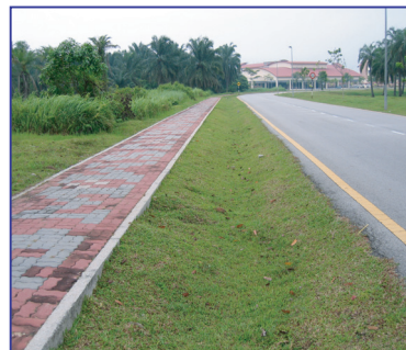
GS6 (Perimeter swale)
