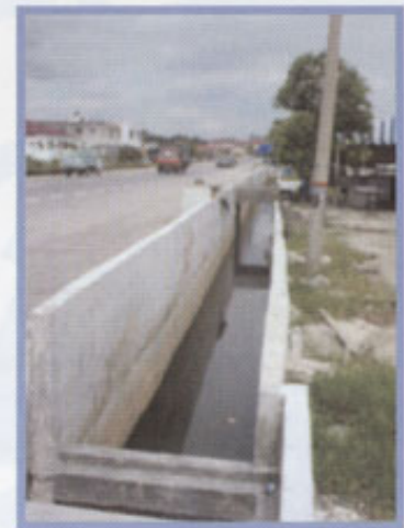
Upgraded Open Drain
