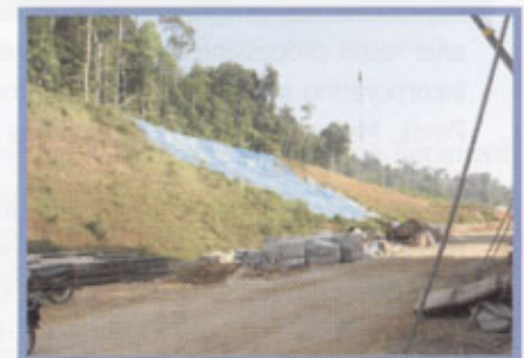
Slope Protection Measure
