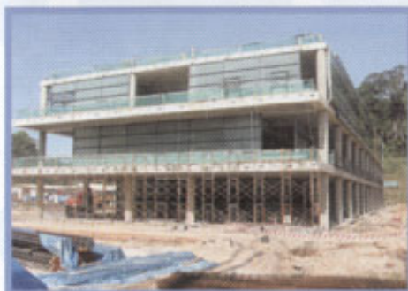
Building In Progress
