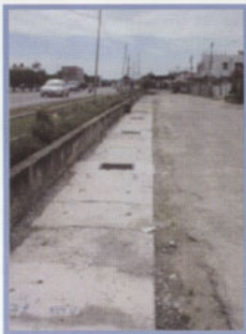
Upgraded Covered Drain
