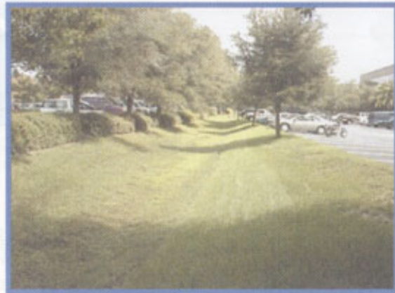
Typical Swale After Construction
