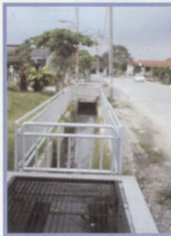
Upgraded Open Drain
