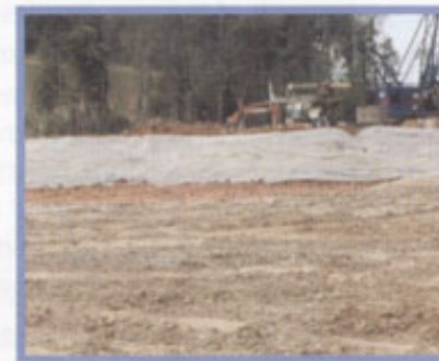
Erosion Mitigation Measure
