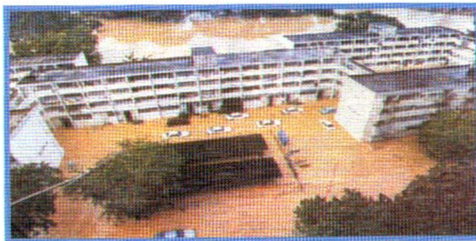
Fig. 2 Pari River overflow during flood on 19th Nov 1997
