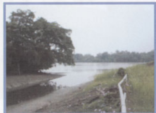
Existing Drainage Condition at Chain Ferry
