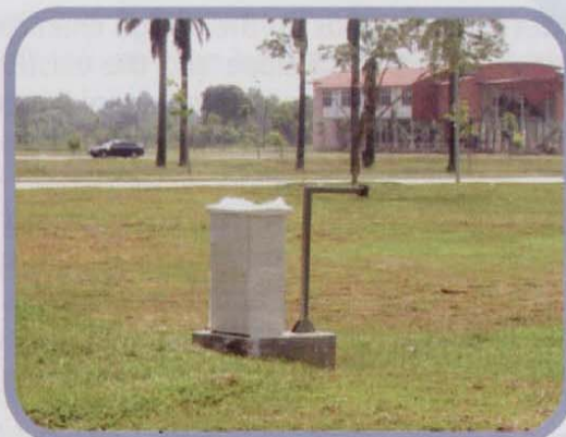
Dry Pond Monitoring Station Site No 1
