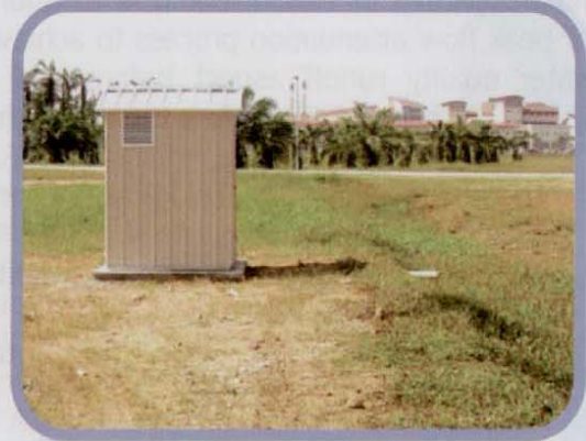
Water Quantity and Quality Monitoring Station No 3 Ecological Swale Type C
