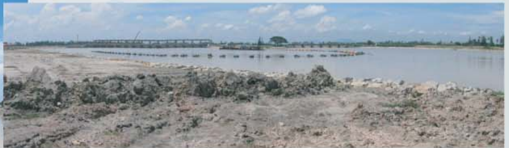
New Barrage Under Construction
