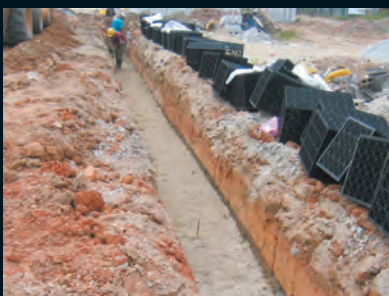
(a) A trench is dug with backhoe and layered with river sand
