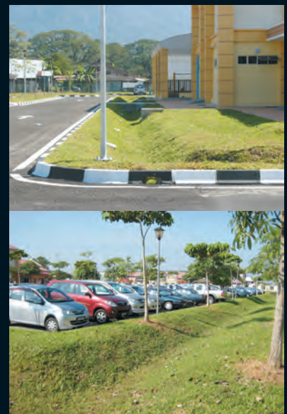
(e) Ecological Swale after Completion
