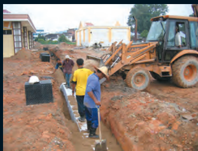
(c) Trench is backfilled with enclosed module buried within
