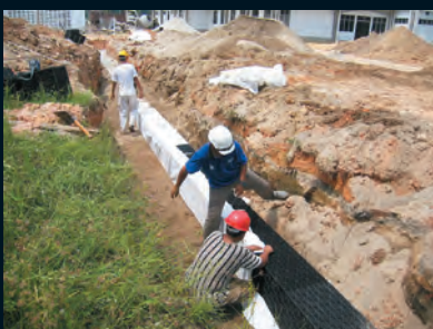
(b) Module is laid in the trench and wrapped in geotextile
