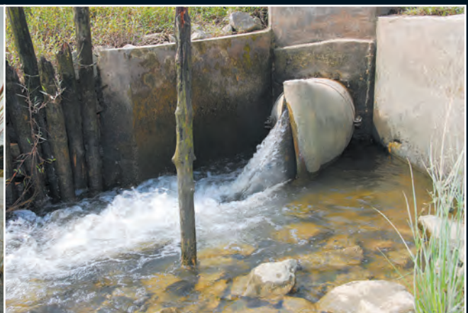
Figure 8 Check valve used to provide flow in one direction only through a culvert
