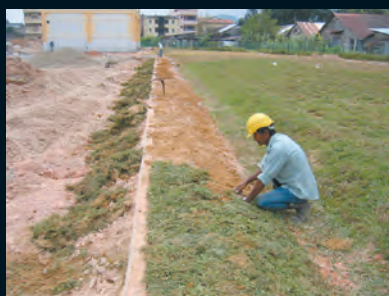
(d) A swale is shaped and topped up with top soil before being turfed
